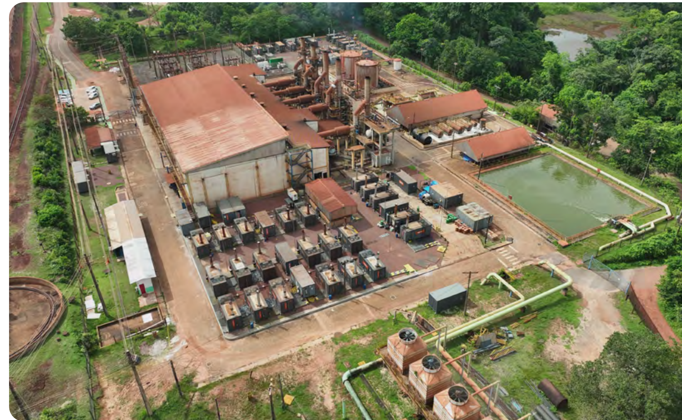
MRN Power Generation Plant
