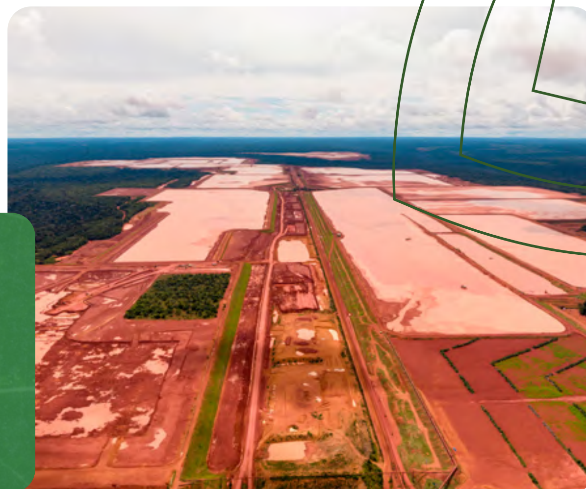
Operational View of the Tailings Disposal System
